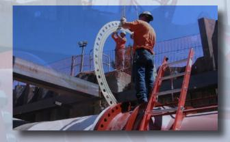
Trojan G-10 gaskets are state-of-the-art, with near zero leakage static sealing and the duplex four seal design further ensures the integrity of the sealing capability. The elastomer sealing
