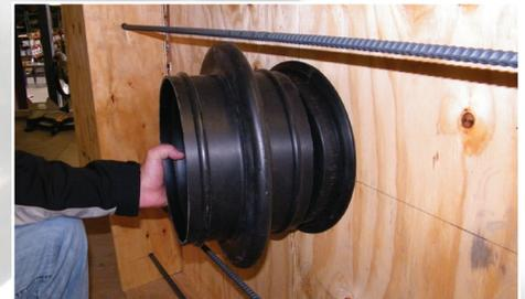
3. Cut the Infinity® wall sleeve  $\frac{3}{4}$ " shorter than the wall thickness (+/-  $\frac{1}{4}$ " ), then insert the sleeve over the locator cap.
