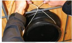
5. Attach the Infinity  $^{\rm I\!B}$  wall sleeve to the rebarusing wire.
