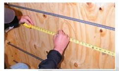
Using a tape measure, pull measurements from the horizontal and vertical positions to locate the center of the Infinity<sup>®</sup> wall sleeve.
