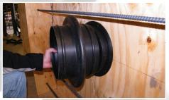
3. Cut the Infinity® wall sleeve ¾" shorter than the wall thickness (+/-1/4"), then insert the sleeve over the locator cap.
