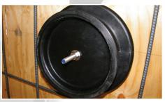
3. Slide second locator cap through (threaded rod\*), use fender washer and fasten nut until locator caps and sleeve are locked in place. Check to make sure sleeve is square to form.
