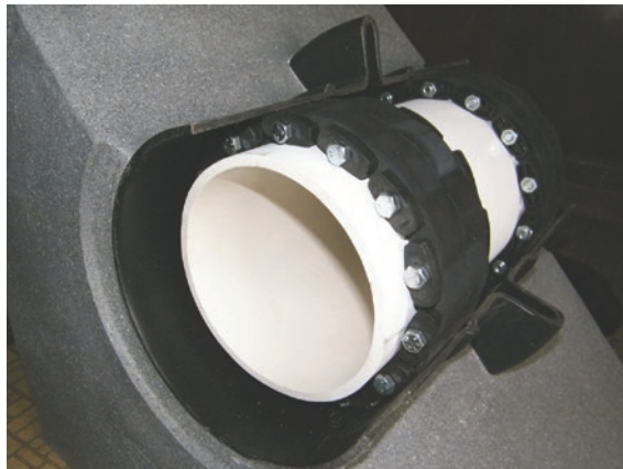
Cut-away view of Infinity® wall sleeve & Innerlynx®
