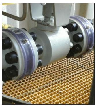
APS presently manufactures Kleerband® Flange Protectors to fit all ANSI flanges 150# series to 2500# series up to 144" diameter. Also available are Flange Protectors to fit API 2000# to 15,000# flanges, API Integral flanges, API obsolete flanges, and AWWA flanges. Available in standard 1 1/2" and 2 1/2" widths. Wider widths available in original design upon request.
